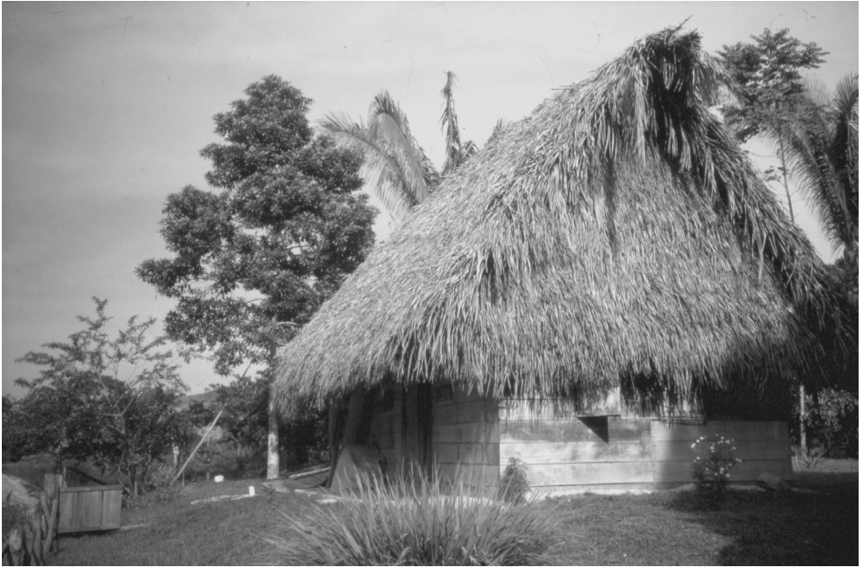
Figure 8.1 The TEA guesthouse in Laguna, Toledo district, south Belize
